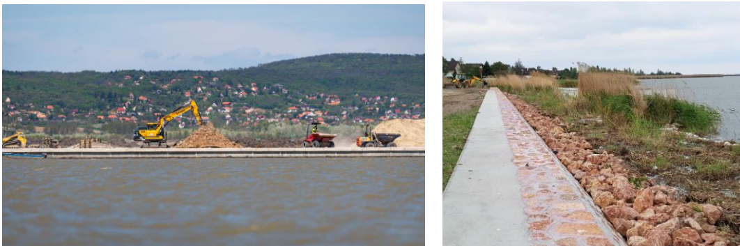
Figure 2.4 A complex renovation project in the shore area of Lake Velence
