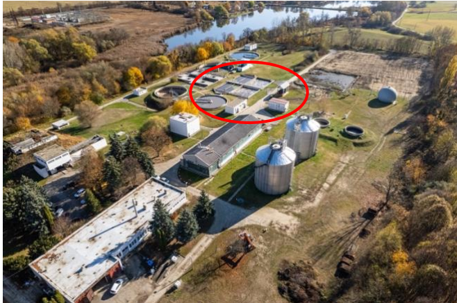
Figure 8: The Gödöllő wastewater treatment plant, with the Isaszeg lake system in the background. Source: own photo
