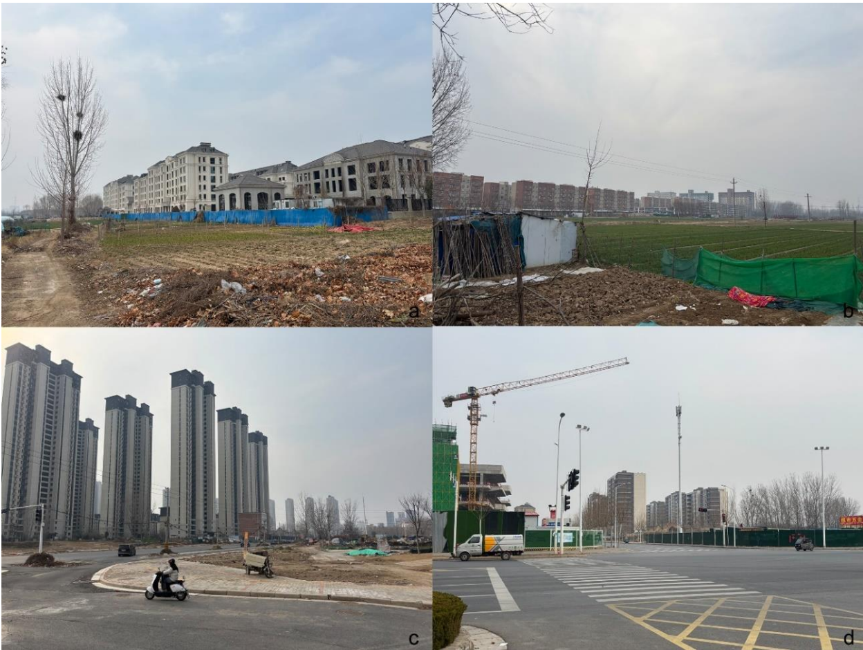
Figure 4.35: Field survey images of Baisha Town.
